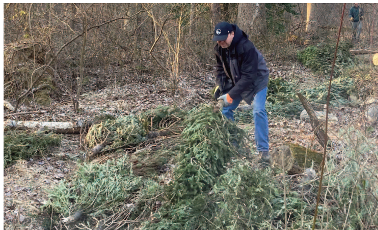
Christmas trees trap sediment when they are laid into swales with their tops pointing up-stream.
